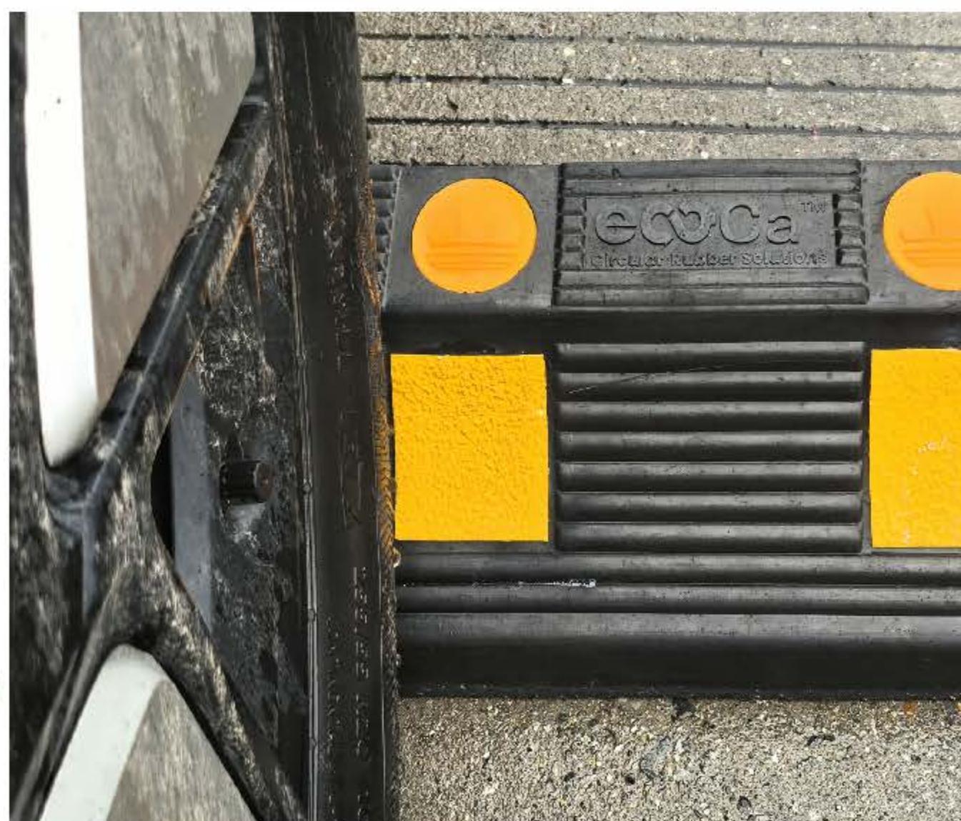
These blocs are not made by gluing still-vulcanized crumb rubber with epoxy or polyurethane (harder to recycle later): They are molded products from devulcanized rubber (yellow tape, to easily remove from the rubber, infinitely recyclable, for much more resistant blocks that last many years)!
